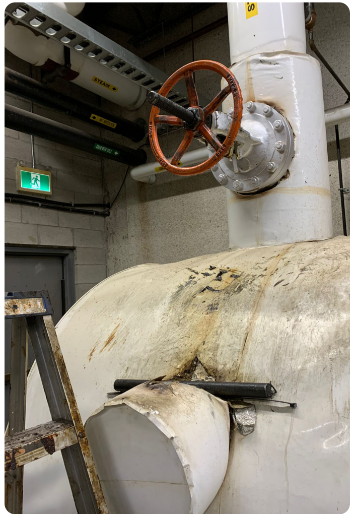
Poorly insulated accumulator steam line
