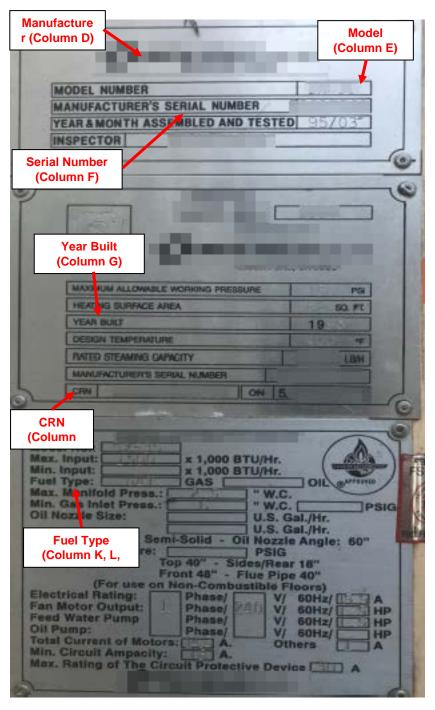
Here are sample boiler plates on a boiler in case you do not know what a boiler plate looks like. Some regulated equipment has more than one of these plates, as per the photos on the left.
