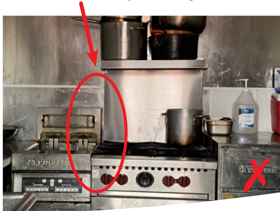
No divider between fryer and range unit
