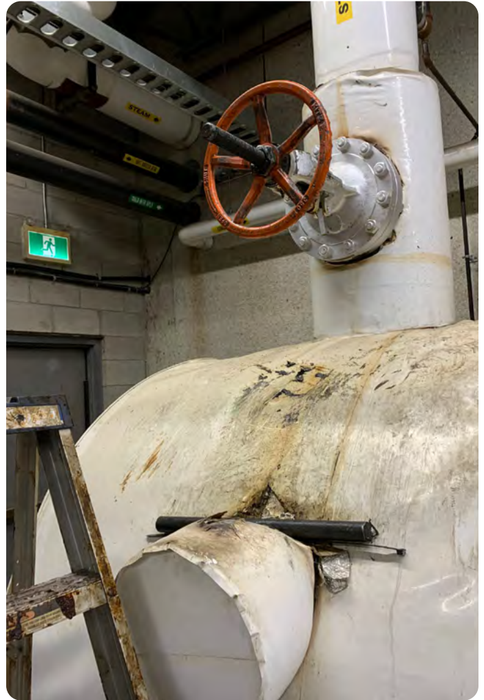
Poorly insulated accumulator steam line
