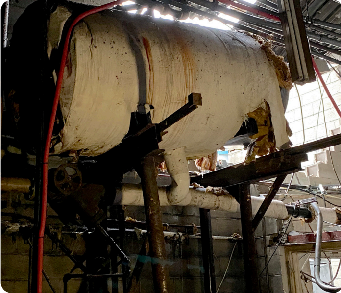
Exploded expansion tank
