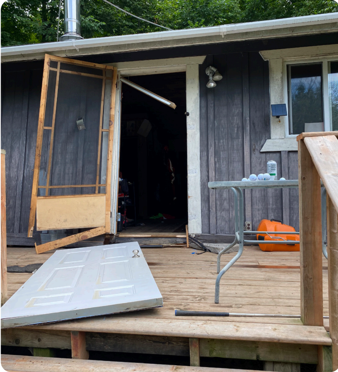
Cottage after explosion
