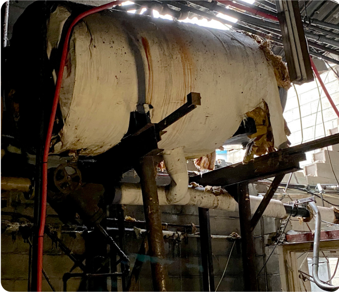
Exploded expansion tank
