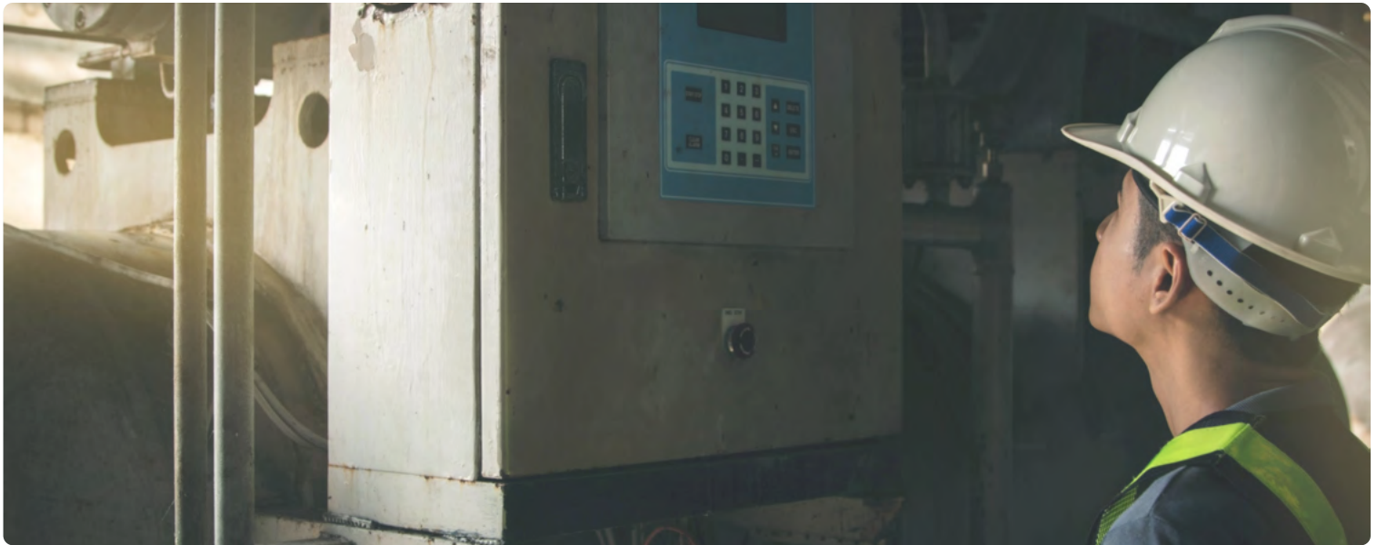
➤ Stock photo: Operating engineer in compressor room
