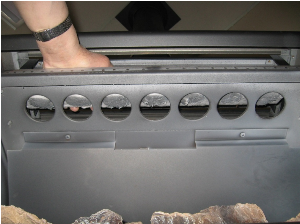
Pressure Relief Openings on Top of Firebox
